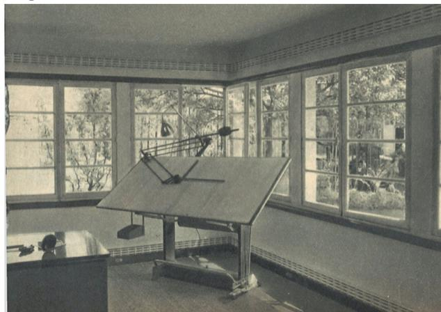
Rubancolor heating tape, manufactured by RAS, girdles not only the ceilings but also the wall bases (1958 Rambert, Le chauffage, Ultimheat Museum)
